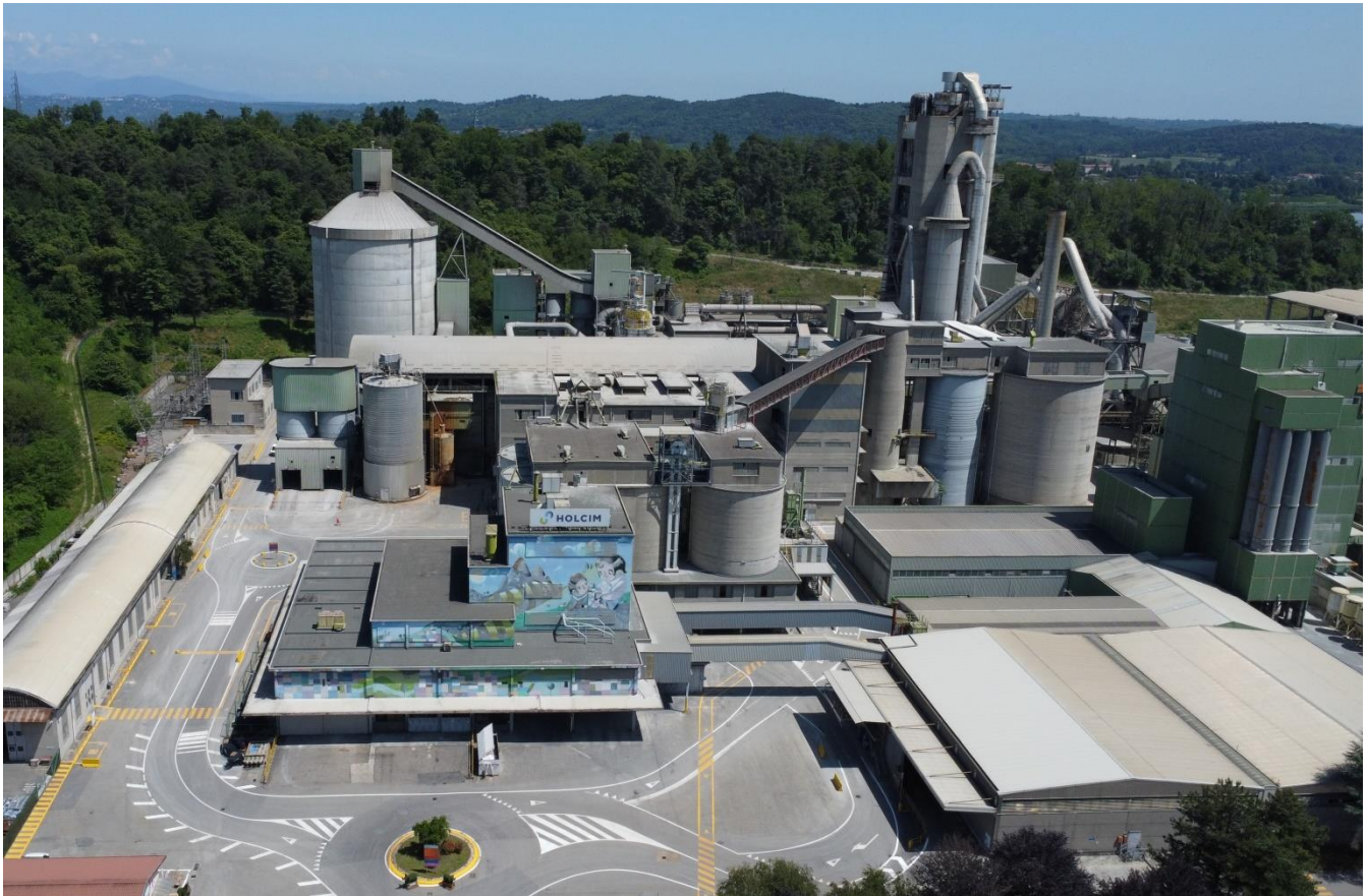
Figura 2. Cementificio Holcim - Ternate
